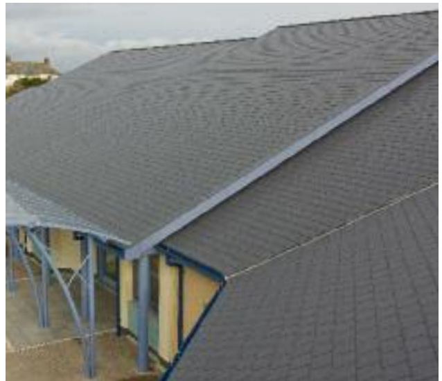
Rivendale Blue/Black, Portfield Special School, Haverfordwest
