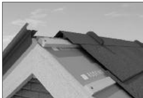
Fig. 8: Nail L/H trim in place.
