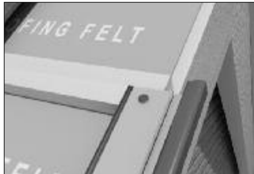
Fig. 2: Cut 15mm in from end of trim.
