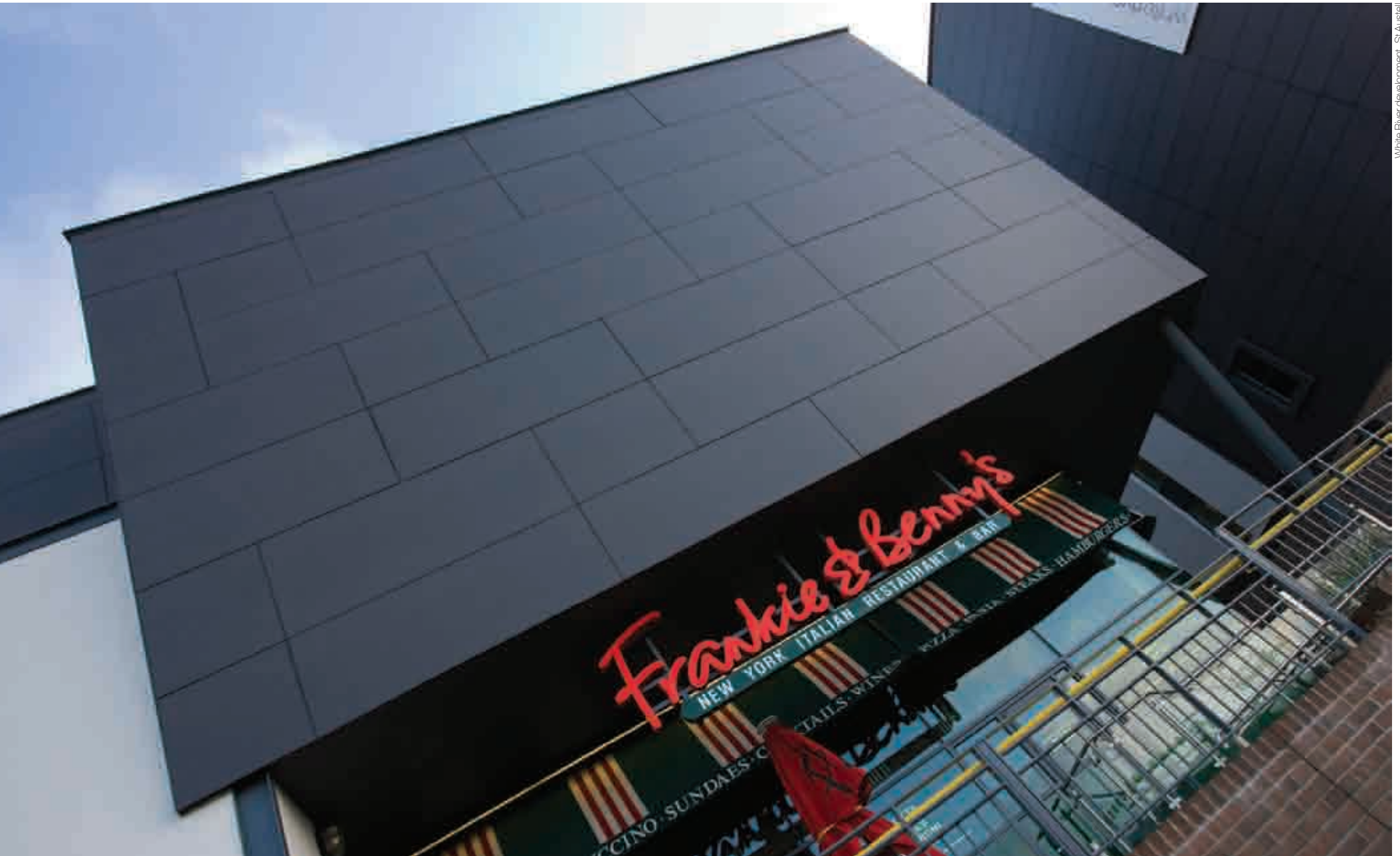
White River development, St Austell
