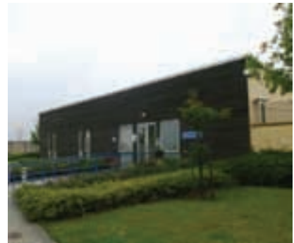
Luton and Dunstable Hospital – prior to overcladding
