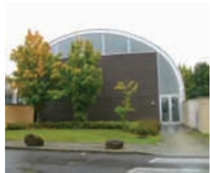
Luton and Dunstable Hospital – prior to overcladding
