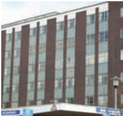
Darlington Memorial Hospital – prior to overcladding
